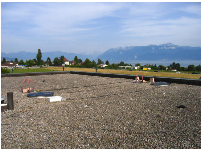
Fig. (2). Setup two (a) and location of the sensors on the rooftop (b).
