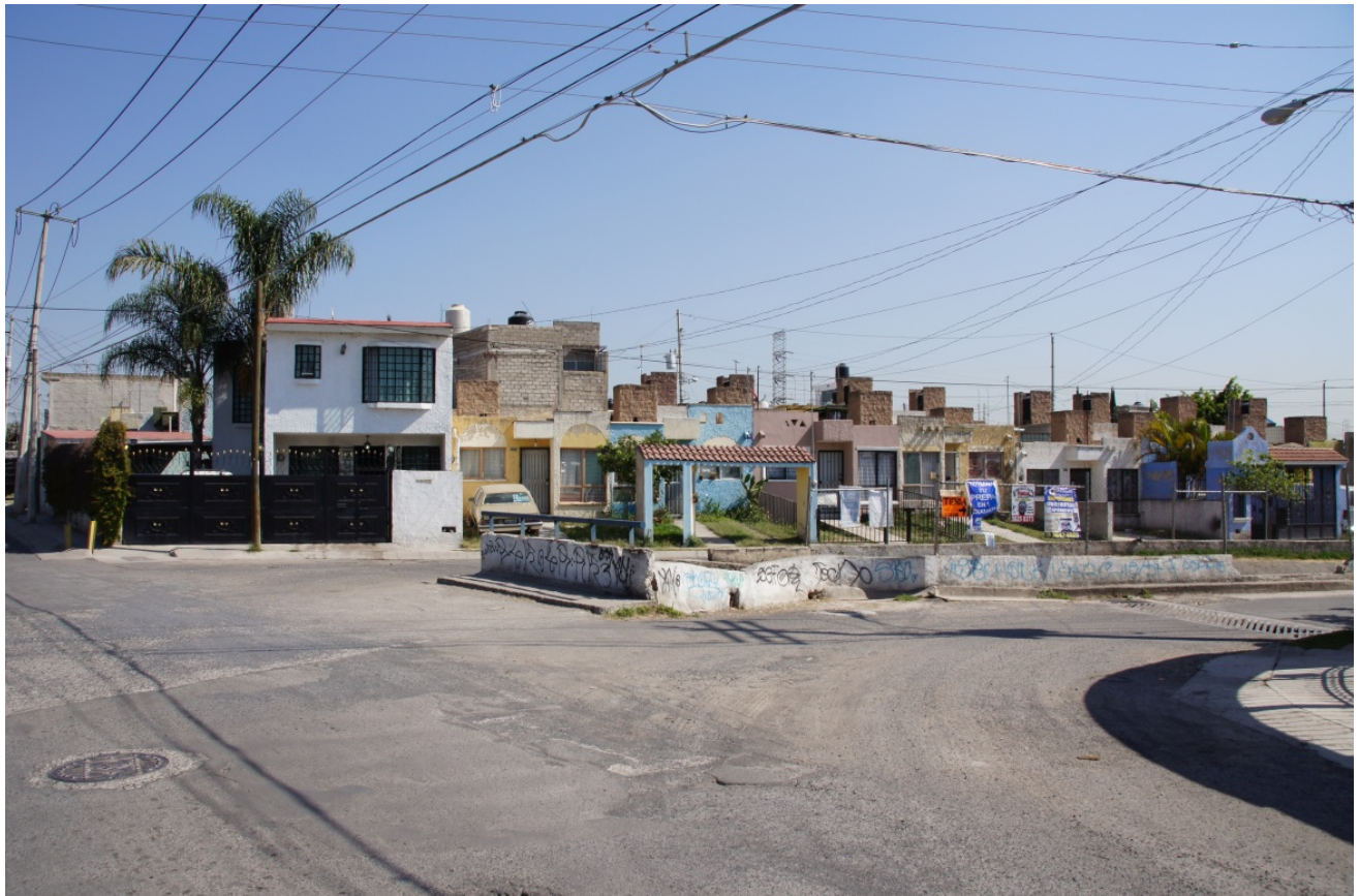
Fig. (9). Open sewer in a peripheral fraccionamiento south of Guadalajara (centre of the picture, small murals building the embankment) (Photograph: A. Budke).
