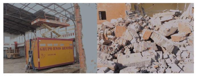
Fig. (3). In the picture on the left, panels containing asbestos are removed as hazardous material by an authorized manager, and on the right, bricks and concrete are treated as non-hazardous and are ready to be crushed and reused.
