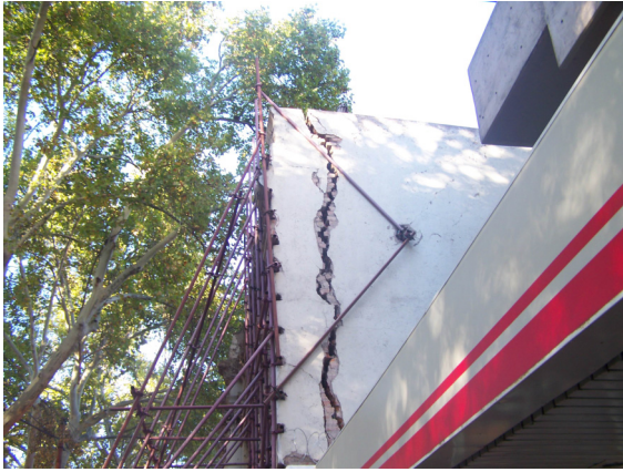
Fig. (10). Cracking of façade (2010).
