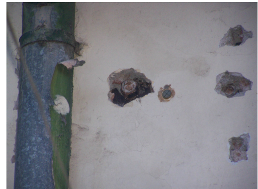
Fig. (8). Detected tighteners.
