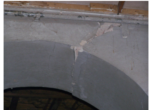
Fig. (14). Cracking of arches.
