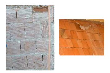
**Fig. (4).** The haphazard nature of the masonry infill matrix to be modelled is clearly seen from these photos taken in Bingol, Turkey, by the author. Where head joints are often missing and bricks are laid in an irregular manner. Clearly, obtaining relevant data for such a material is a challenge.
