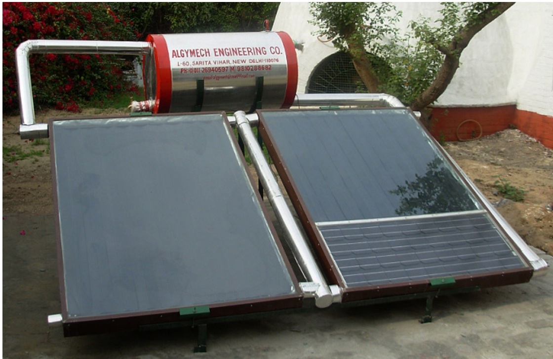
Fig. (1). Photograph of a combined photovoltaic thermal (PV/T) glass to glass solar water heating system.
