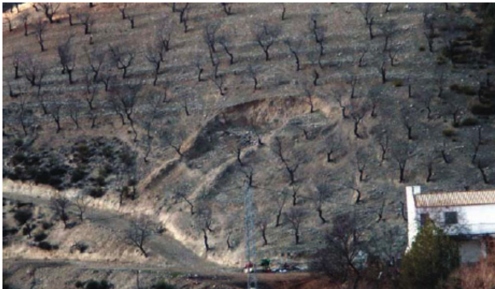
Fig. (5). Small landslide caused by road construction in the detrital source area. Intense human activity in the catchment area covered by the Granada Basin detrital sediments are largely responsible for the huge volume of sediment supply in the transverse detrital system.
