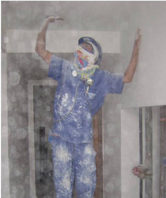
Fig. (3). Sanding the ceiling for paintwork.
