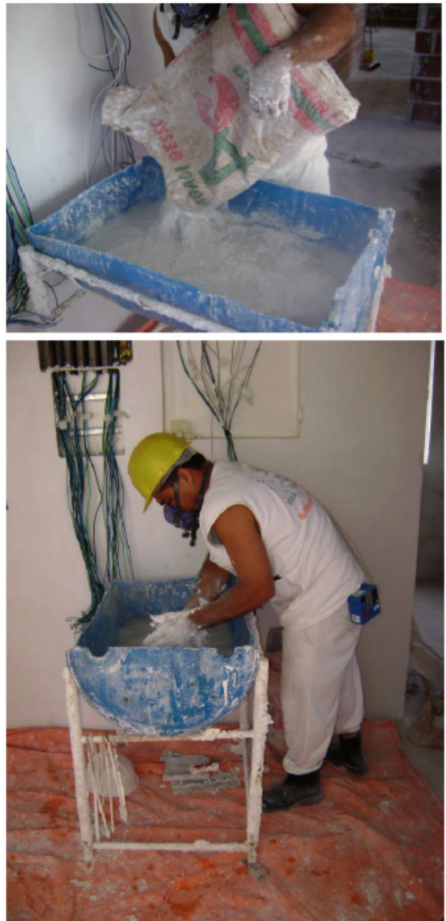
Fig. (2). Preparation of plaster (top: unbagging the plaster powder; bottom: preparing the plaster paste).
