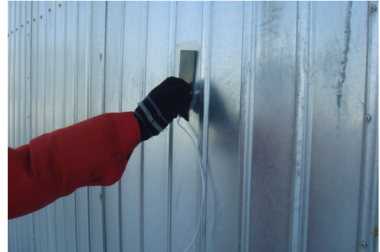
Fig. (3). Installation of heat flow meter probe.
