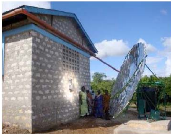
Fig. (6). Field-scale solar concentrator installed at Kinango, Kinango District, Kenya.
