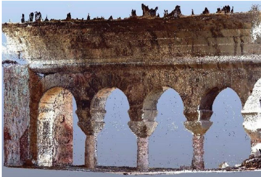
Fig. (6). An example from the point cloud data of the structure.
