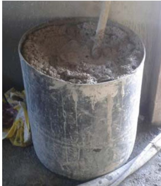
Fig. (17). Packaging of waste from equipment cleaning.
