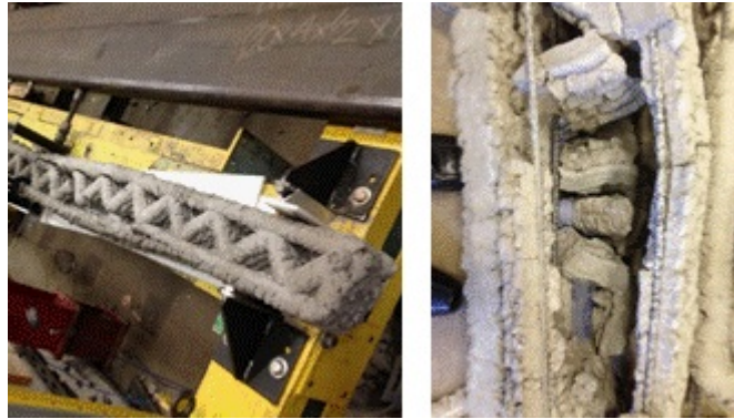
Fig. (15). Mode of failure for beam 5DR-B-0: tension failure, debonding between basalt rebar and concrete, and shear failure at nodal points.
