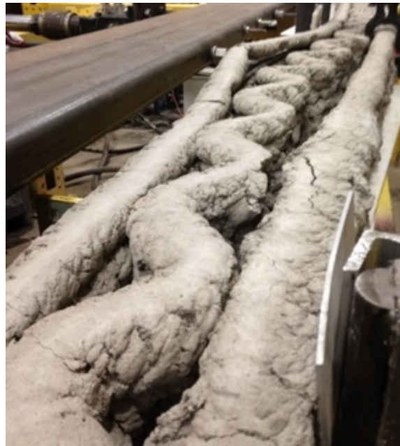
Fig. (17). Mode of failure for beam 6DR-S-6B: shear failure at nodal points, debonding between steel rebar and concrete, and tearing of basalt mesh.
