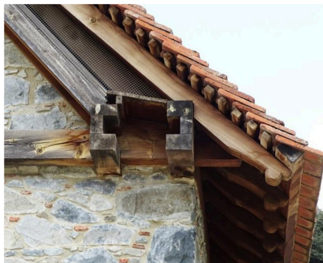
Fig. (5). Church of Panayia at Moutoullas village. Detail of the connection between the timber roof and the south wall (Photo M. Pelekanos).
