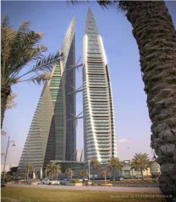
Fig. (1). The three parallel wind turbines are able to generate between 1100 and 1300 MWh per year, which will amount to approximately 11 to 15 per cent of the office tower's electrical energy consumption.
