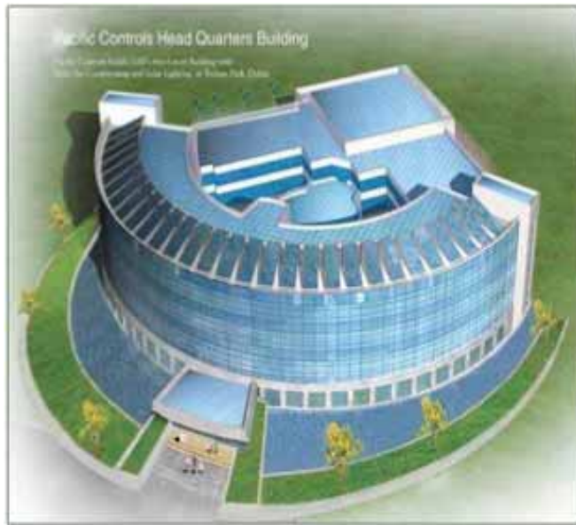
Fig. (9). The 1st LEED Platinum rated Green Building in the UAE. Pacific Controls Headquarters in Techno land, Dubai. The Building uses thermally Efficient roofs, walls & windows, HVAC systems & efficient electrical lighting strategies that capitalize on daylight and HVAC system incorporating solar air-conditioning using absorption chillers.
