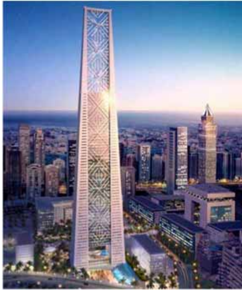
Fig. (11). The lighthouse in Dubai is a 400m high; 66-storey commercial office tower; three 29m diameter, 225 KV wind turbines; 4000 PV spandrel panels; 84,000 m 2 of commercial space as well as basement and podium parking, convention centres, retail, environmental visitor centre and a park connecting to the DIFC central spine.
