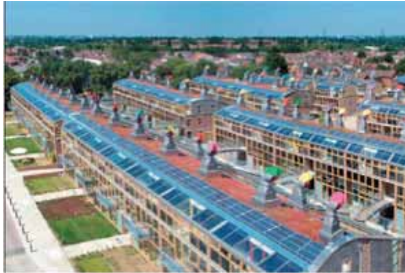
Fig. (17). The Bedzed, zero energy (gallerid apartments in Great Britain); a pilot project integrating sustainable technologies.
