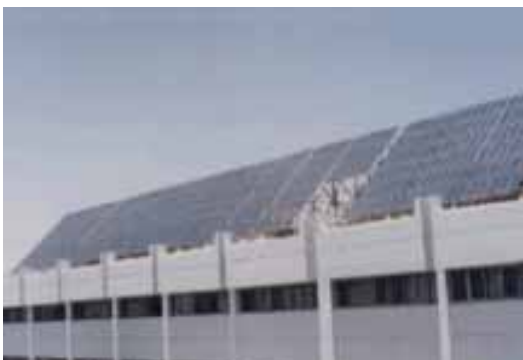
Fig. (12). Kuwait English School (Salwa): The First BIPV in the Middle East (1984).
