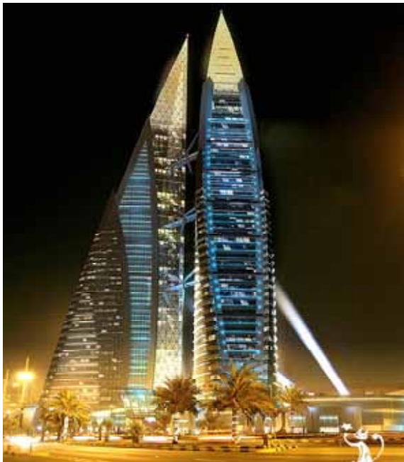
Fig. (2). The three parallel wind turbines are able to reduce the carbon emission terms this equates to an average of 55,000 kg of CO 2 (UK electricity basis).
