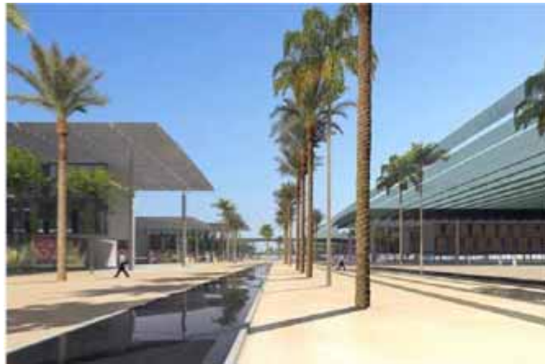
Fig. (6). A walk way at Euro University showing major PV covered area providing shade and producing electricity.
