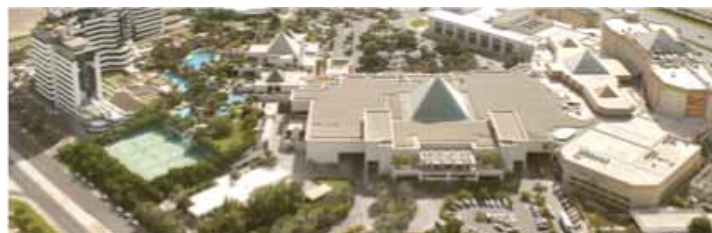
Fig. (8). The Wafi City District Cooling Chiller Plant DCCP ONE.
