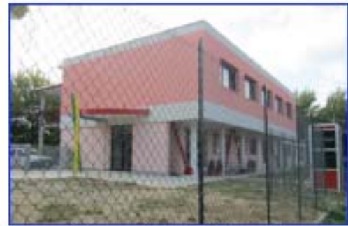
Fig. (19). View of the building after the completion of the retrofit and architectural renovation works.
