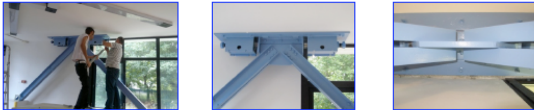
Fig. (18). Final half-stroke positioning of a spring-damper, and views of the same DB panel.
