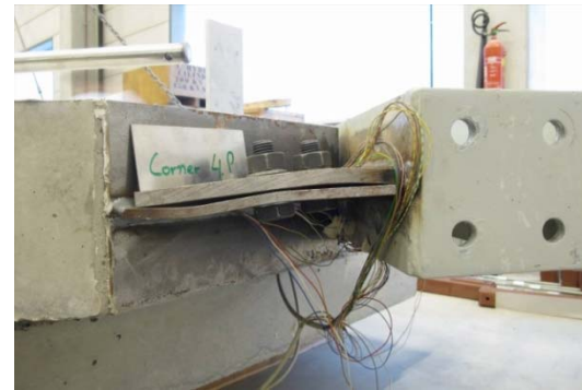
Fig. (14). Out-of-plane deformations in anchor and gusset plates of FPC3.
