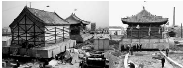
Fig. (8). The track sharing- monolithic movement method.
