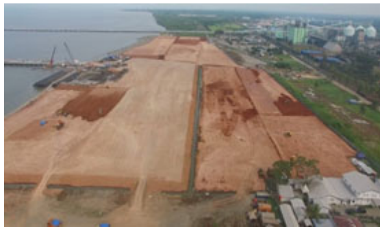
Fig. (2). Photograph of the embankment area of the case study.
