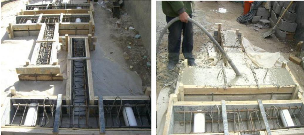
**Fig. (2).** Specimens preparation.
