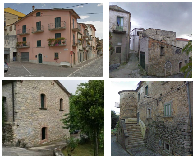
Fig. (3). Street views of the characteristic building typologies within the historical centre of Baranello.
