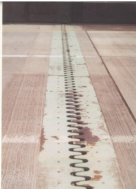
Fig. (11). Typical expansion dam.
