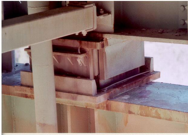
Fig. (14). Close-up view of the sliding bearing.
