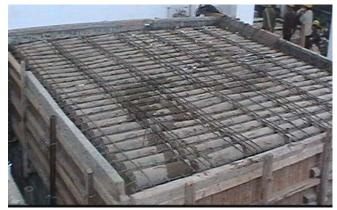
Fig. (1). Stiffening-ribbed-pipe girderless floor.
