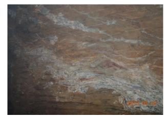
Fig. (19). Slurry veins exposed by excavation.
