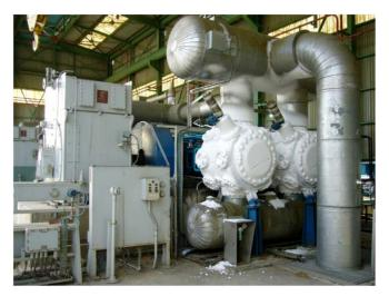
Fig. (2). Horizontal type BOG compressor.
