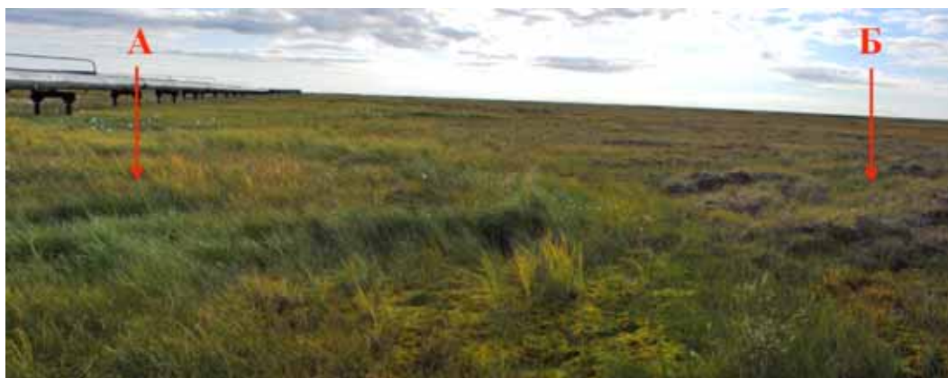
Fig. (10). Thermocarst bogs along gas pipeline (A) and nearby undisturbed background ecosystem (B).
