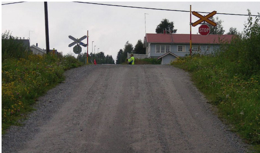
Fig. (7). Steep approach to a level crossing.
