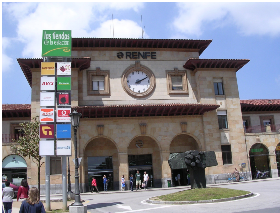
Fig. (1). The renewed rail station in Oviedo. Source: self-made.
